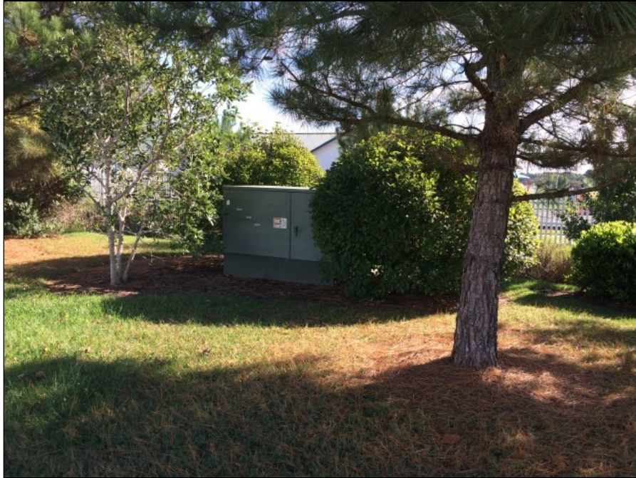
3 - View of the pad-mounted transformer located on the eastern portion of the property
