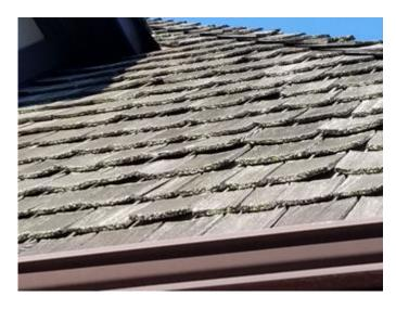
Issue The roofing is loose. This permits water penetration.
