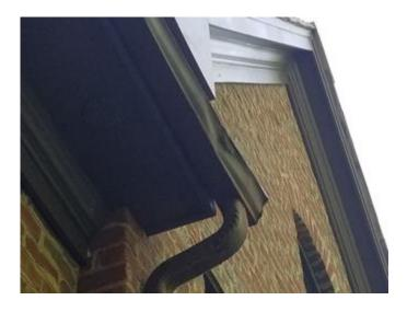
Issue The gutters are loose. This affect proper water control and permits water intrusion and deterioration.
