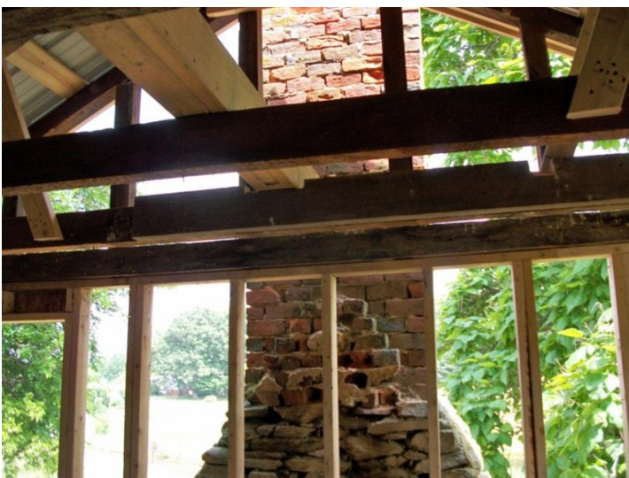
South end framing, drainage over inverted brick 'V' needed to be addressed, 2011
