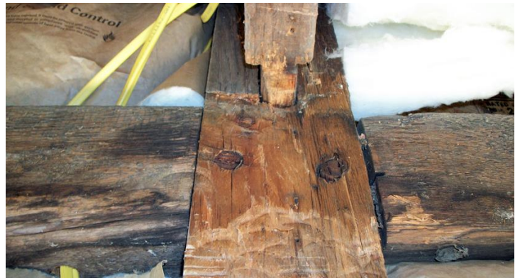
Mortise-tendon joint & pegs
