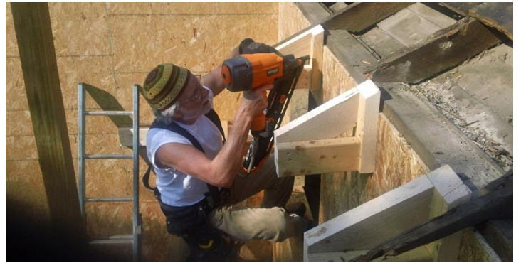
David Brown rebuilding Addition roof overhang
