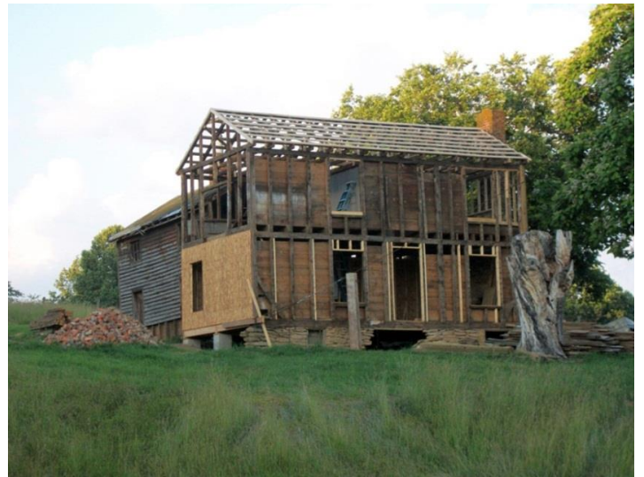
New roof supports and purlins, 2011
