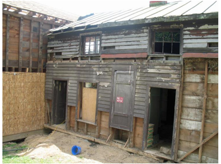
Addition sitting on ground; door with red sign went from outside to upstairs
