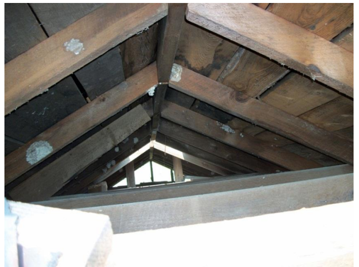
Oak underlayment, Addition roof, 2011
