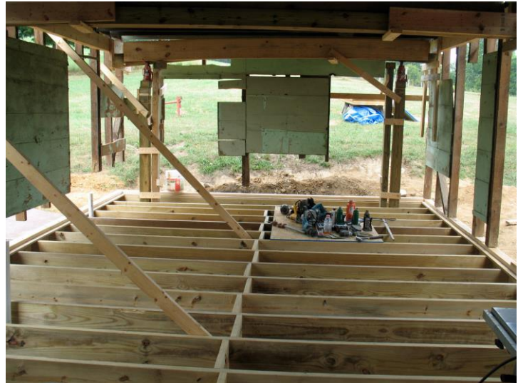
Addition new floor system and sill
