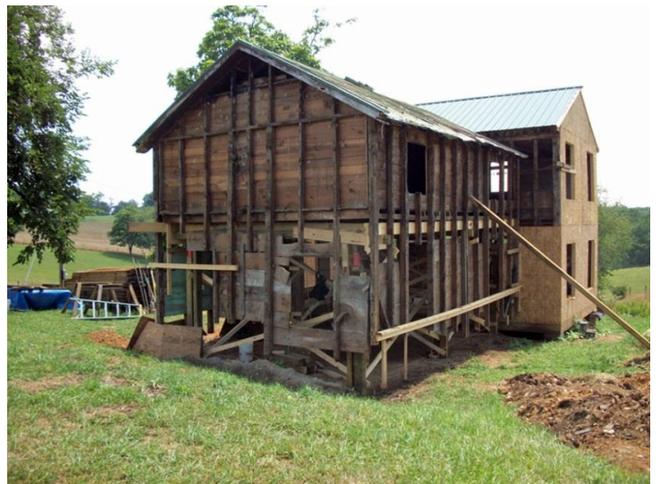
Addition jacked up 18" above ground, freestanding, 2011
