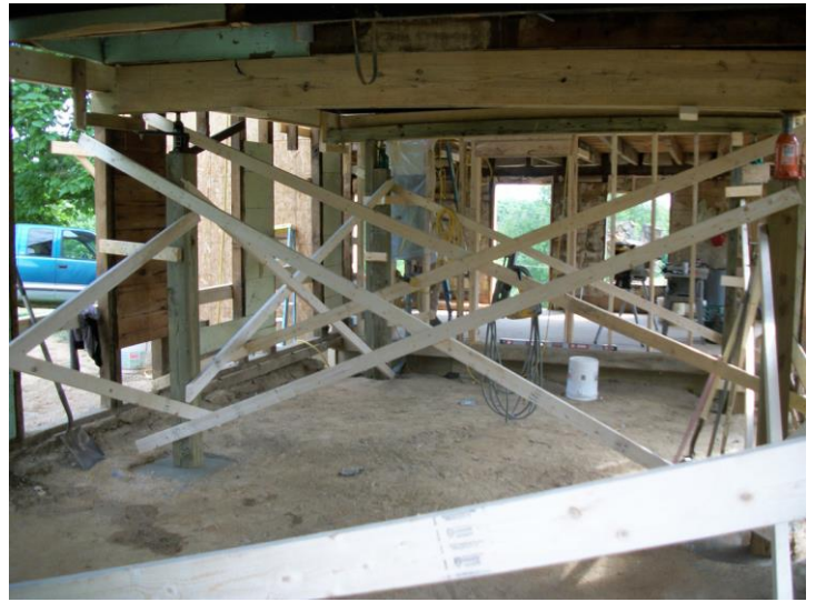
Addition braced to jack
