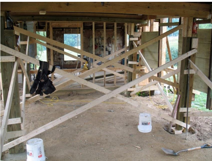
Addition braced and jacked up after floor, internal walls, 10" of dirt removed, 2011
