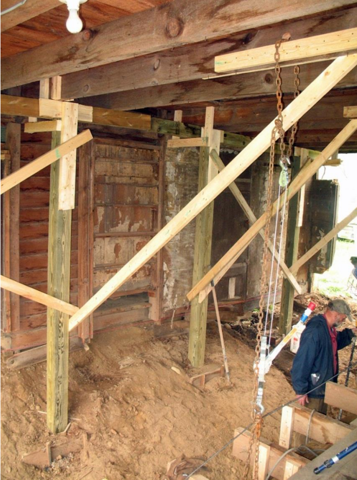
Original part of house jacked up, half of floor suspended from ceiling joists, center support for floor being built, 2011
