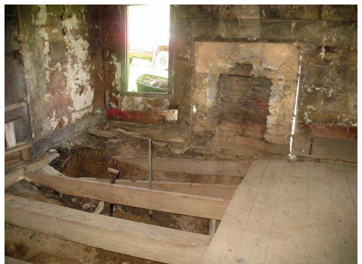
Collapsed Southeast end of Living room in 2011 – sill beam of original cabin in foreground
